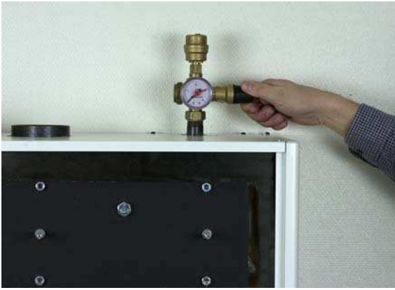
1. Turn the safety valve a few times a year to check the operation of the safety valve.
